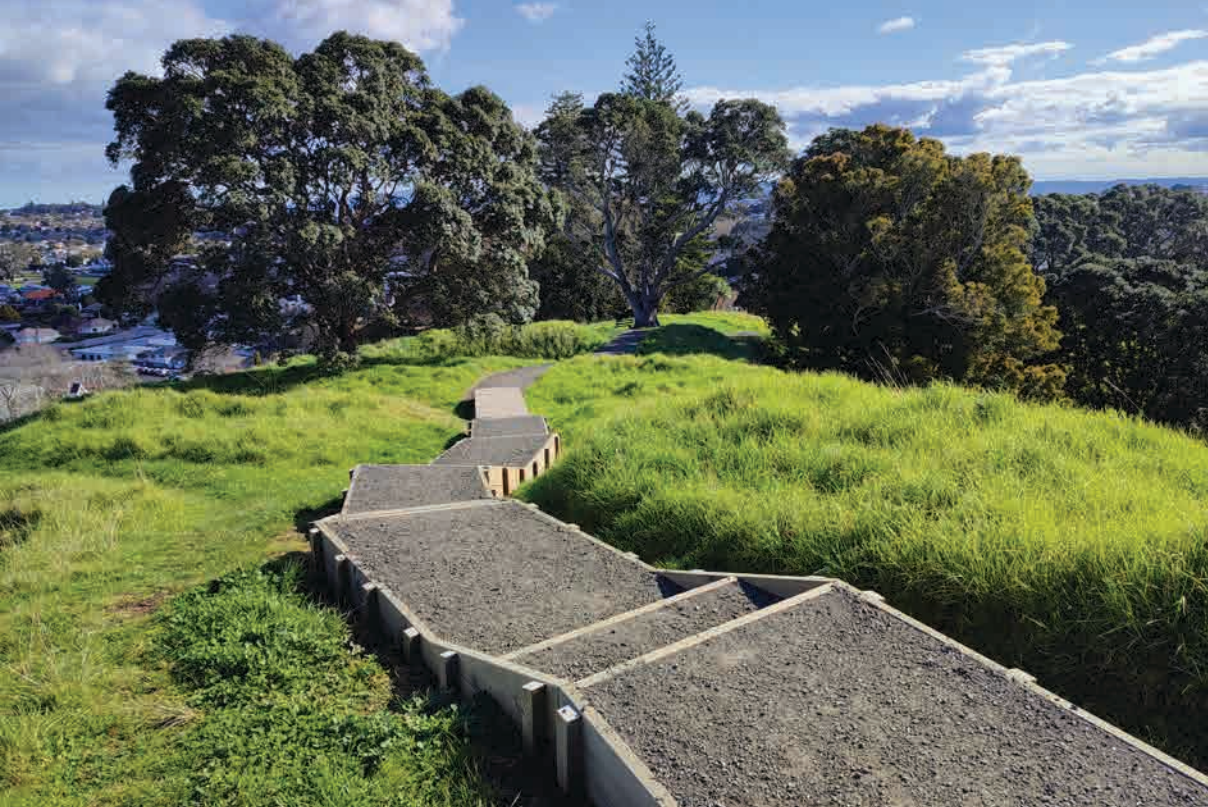
Figure 7. View of board walk going over ditch and boxed steps beyond.
