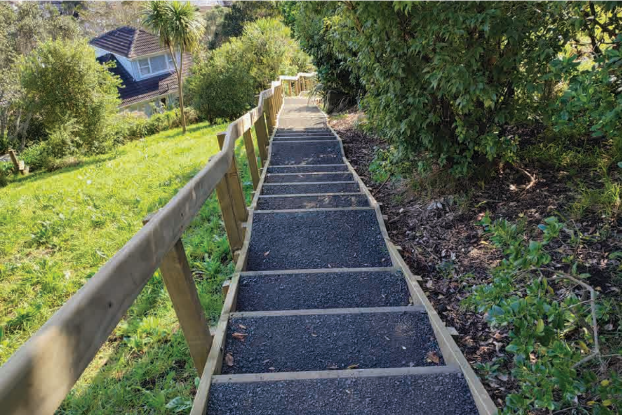
Figure 8. New boxed steps from Belvedere Road entrance.
